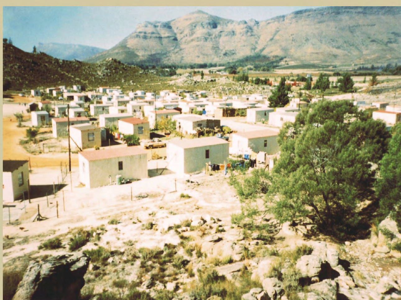
Figure 1. The high density housing suburb of Op-die-Berg Koue Bokkeveld. A large number of leaks were found here.
