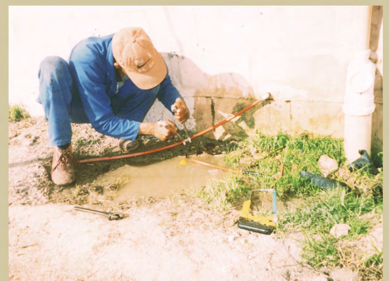
Figure 3. A leak is repaired at Op-die-Berg.
