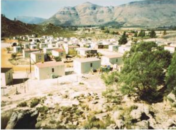
The high density housing suburb of Op-die-Berg Koue Bokkeveld. A large number of leaks were found here.
