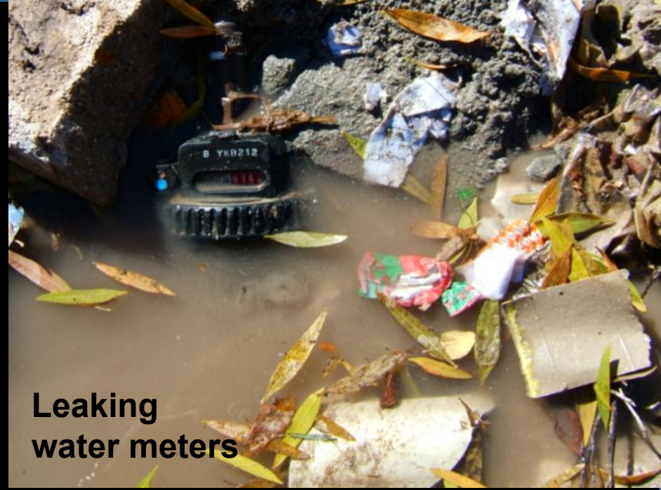
Extreme cold bursts pipes & taps
