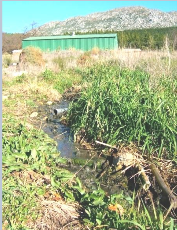
Sewerage treatment plant overflowing into a tributary to the Olifants River
